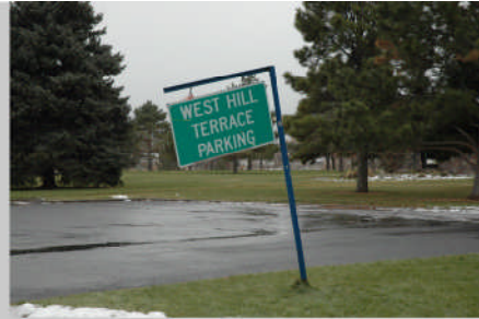
Leaning Sign Post
