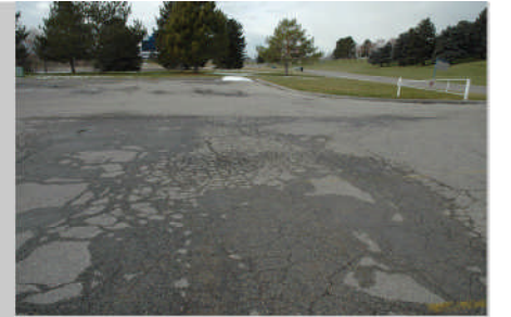
Pavement Cracks
