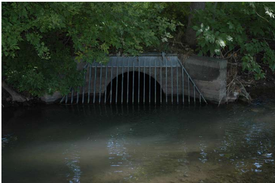
Figure 3. One of several storm drain outfalls draining to Parley's Creek.
